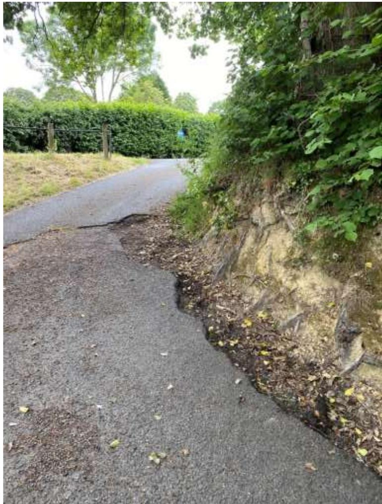
**Fig 1. Potholes and damage to road edges: White's Lane**
