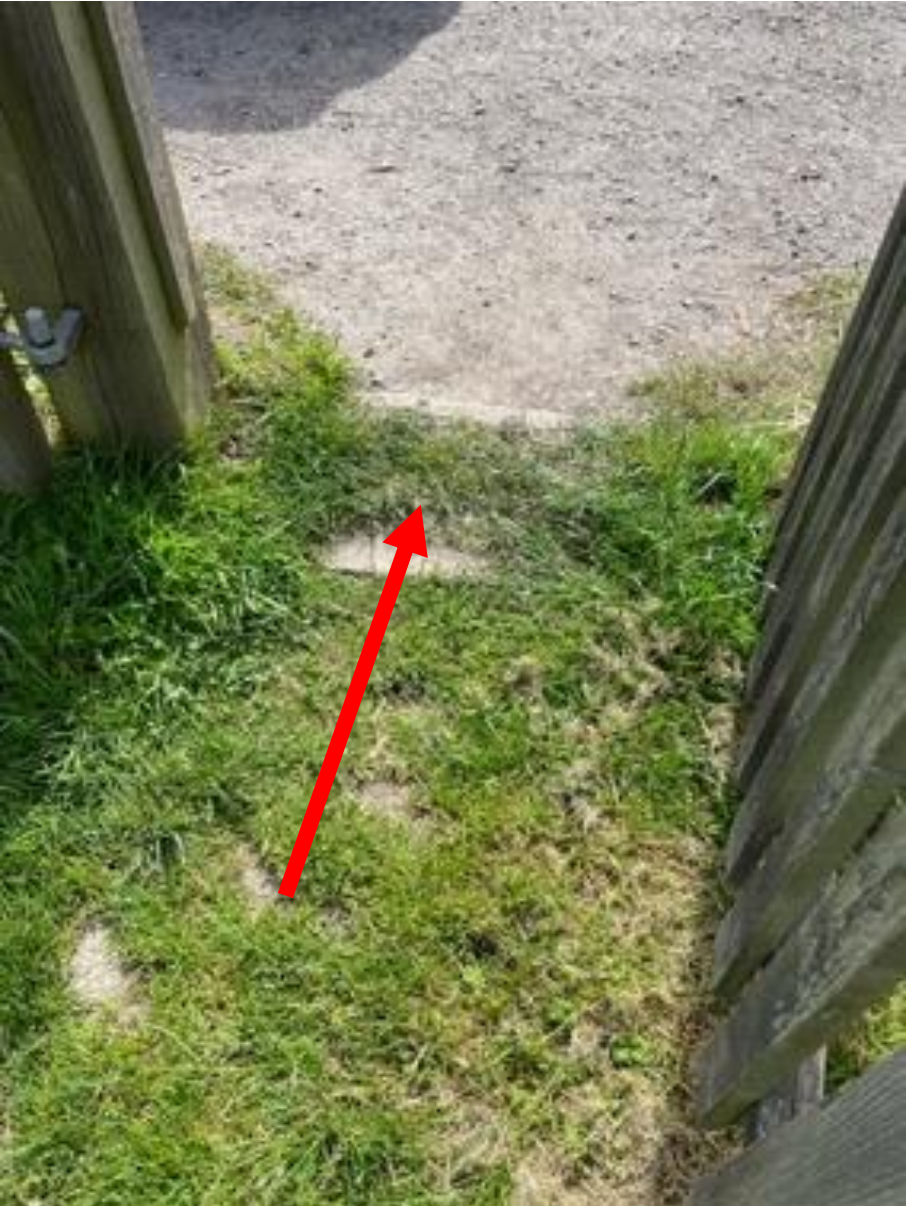
Entrance gate raised edge
