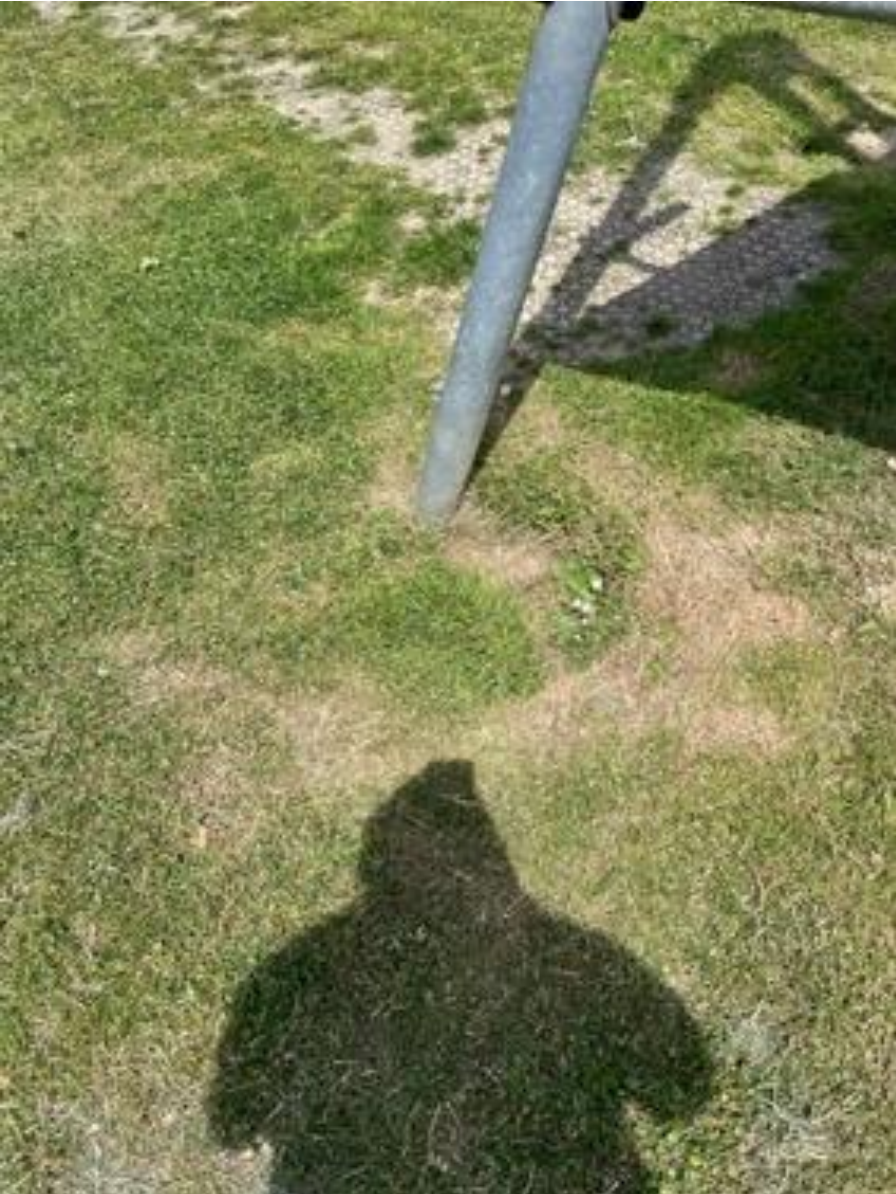
Potholes around zipwire base
